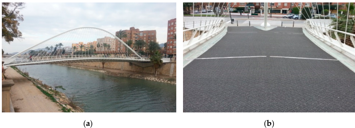
Figure 1. Jorge Manrique footbridge. (a) Longitudinal view of the structure and (b) view of the vinyl flooring installed on the footbridge.
