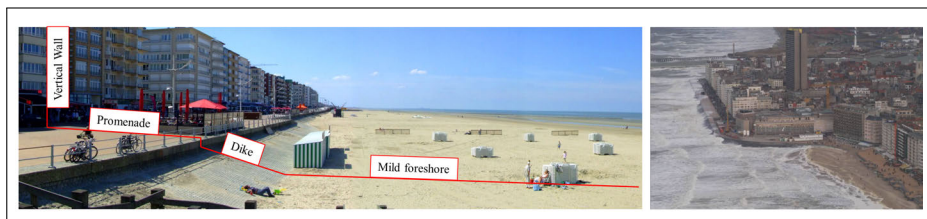
Figure 1.3: Storm water level reaching the dike in Ostend, Belgium (right figure). Before the beach nourishments were carried out starting from 2007 (Van Doorslaer et al., 2017). Typical coastal set-up for the Belgian coastline (left figure). With the soft-structure mild foreshore, followed by the hard-structure dike, promenade and wall (photo by Nicolas Milot).
