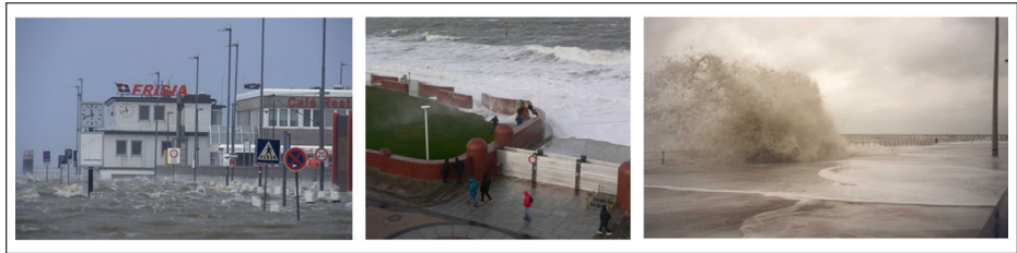
Figure 1.4: Flooding of the harbor in Norden (Germany) during a storm surge (left figure). Wave overtopping of the dike and impact at coastal structures on the barrier island Norderney (middle figure). Overtopping wave splash at the Belgian coast before the nourishment starting from 2007.
