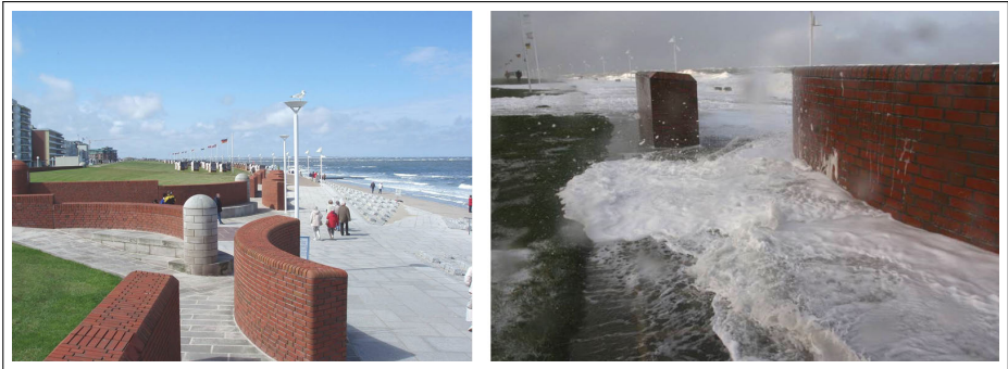
Figure 1.5: Storm walls on the barrier island Norderney during regular conditions (left figure) and during a storm surge with overtopping bore-induced loads on the wall elements (right figure). The storm fotos were taken 09.11.2007 (source: NLWKN).
