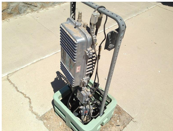
Figure 1-24: An amplifier on a trunk line in a small street cabinet.
