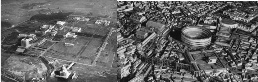
Fig.7 Aerial view of E42 still in construction, 1953.
