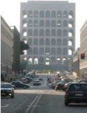
Fig.3 The front façade of the Palace of Italian Civilization (Guerrini, La Padula, Romano, 1938), author’s photograph 2004.
