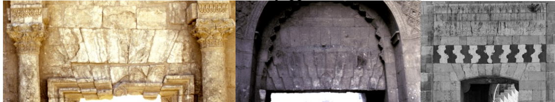
Fig. 4 Rusāfah, city wall, north gate, VI cent.; Bāb al-Futūh, Cairo, 1087; Aleppo gate to the citadel, XVI cent.
