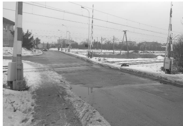
Figure 4. Railway and road crossing II.
