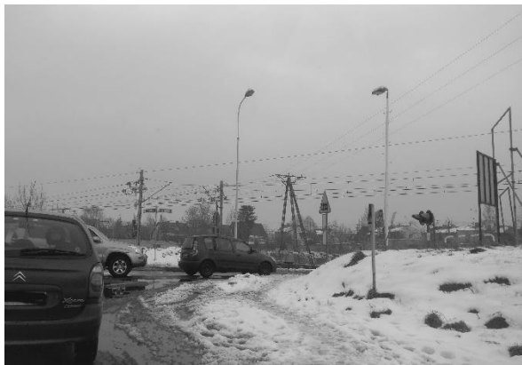
Figure 3. Railway and road crossing I.
