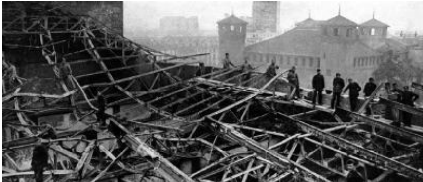
Figure 1.13 The theater cover collapsed because of the flames.
