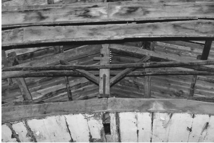
Figure 2. 16 Covering with truss – Garibaldi Theatre Palermo.
