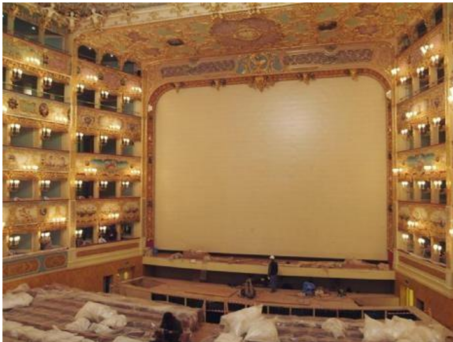
Figure 2. 24 Single leaf fire safety curtain with single leaf of the Teatro "La Fenice" in Venice. Ref; available on site teatrolafenice.it
