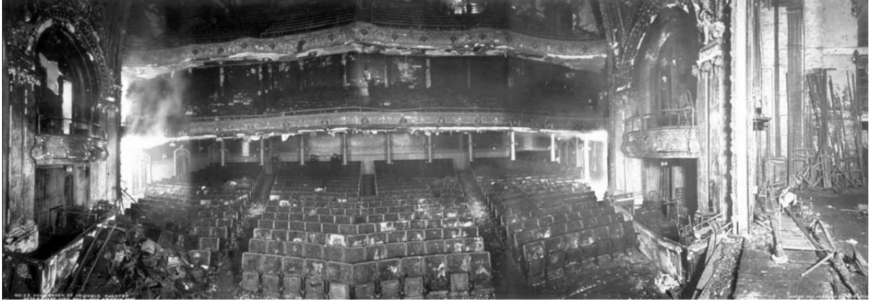
Figure 1. 10 Photograph of the interior of the Chicago Theater after the fire. Ref; The Chicago Daily Tribune. (31, December,1903)
