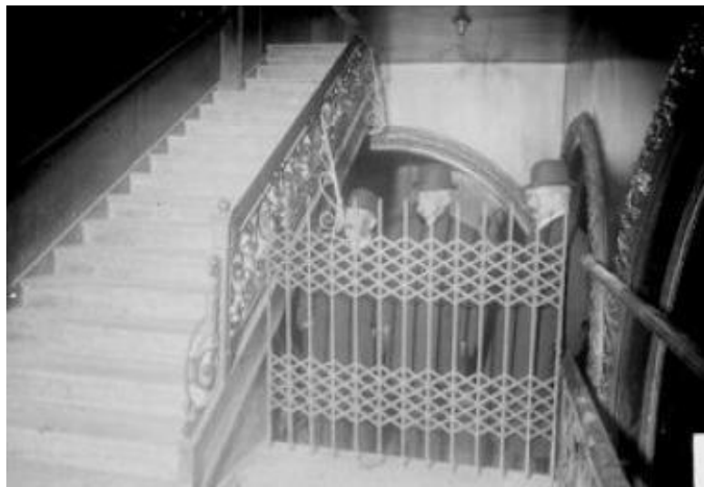
Figure 1.11 One of the locked exits that prevented the escape from the theatre. Ref; William Paul Gerhard, "Theatre fires and panics: their causes and prevention", John Wiley & Sons, 2009
