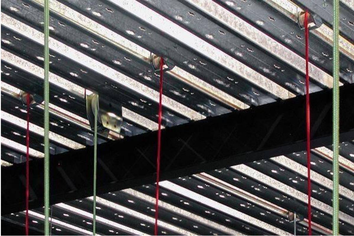
Figure 2.13 Detail of a steel trellis with a system of shots.
