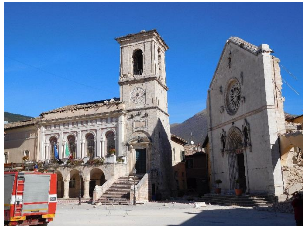
Figure 2. Civic Tower and the façade of San Benedetto Basilica.
