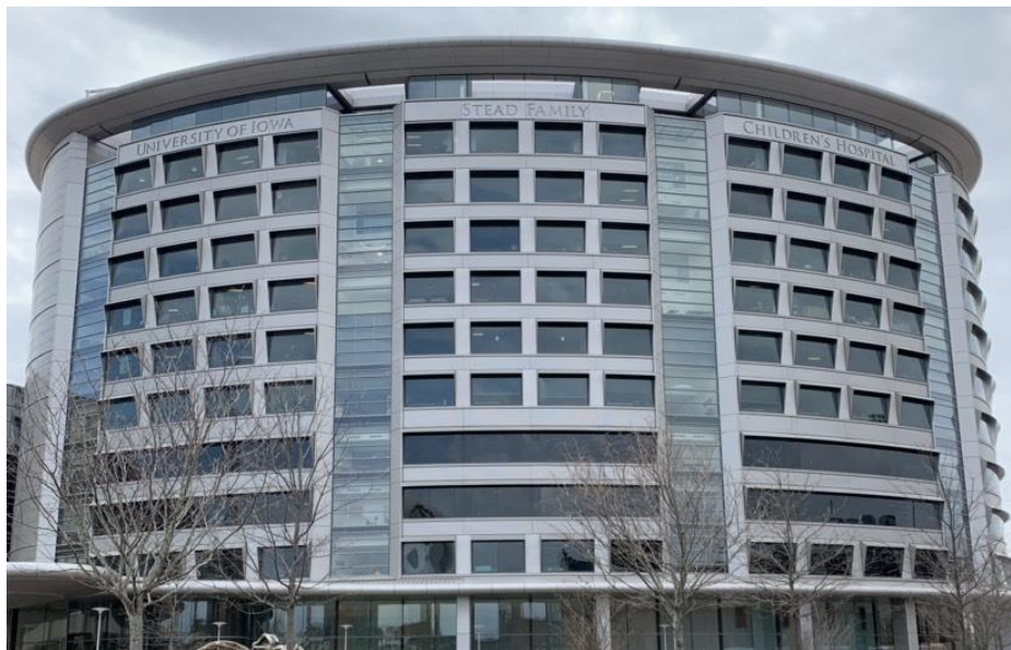
Figure 1: This image shows the 12-floor tower that makes up the Stead Family Children’s Hospital. The Child Psych Unit is located in the main hospital.
