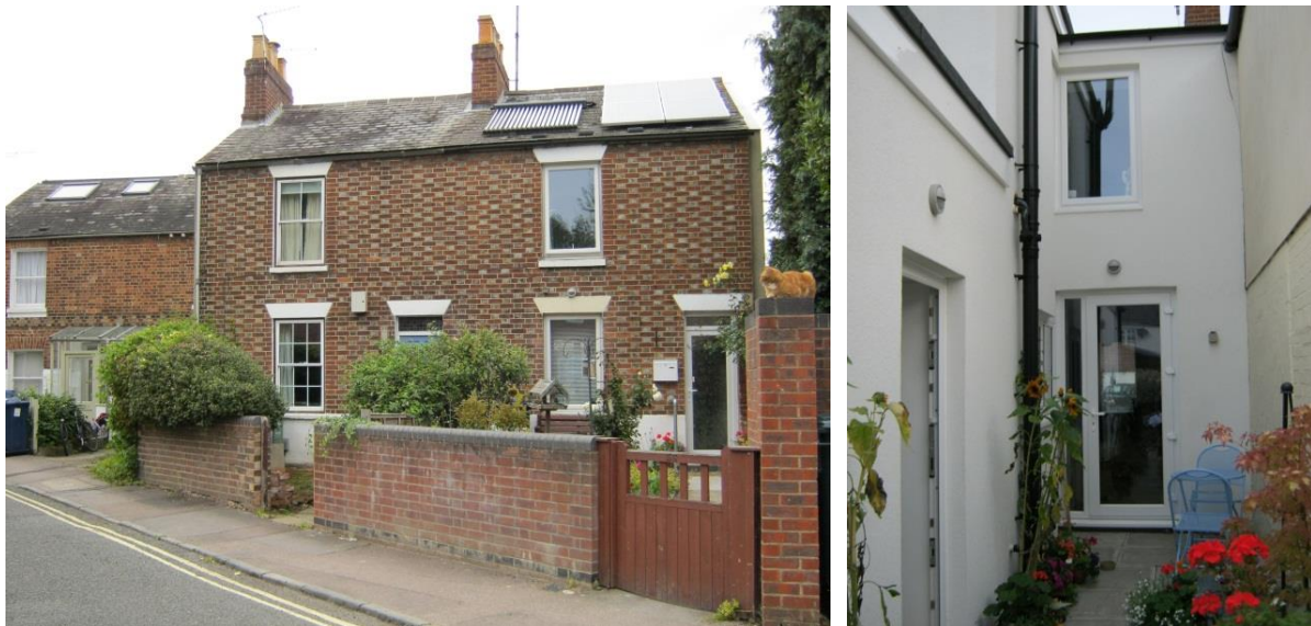
Figure 1 Victorian dwelling post-retrofit – front (left) and rear (right) facades
