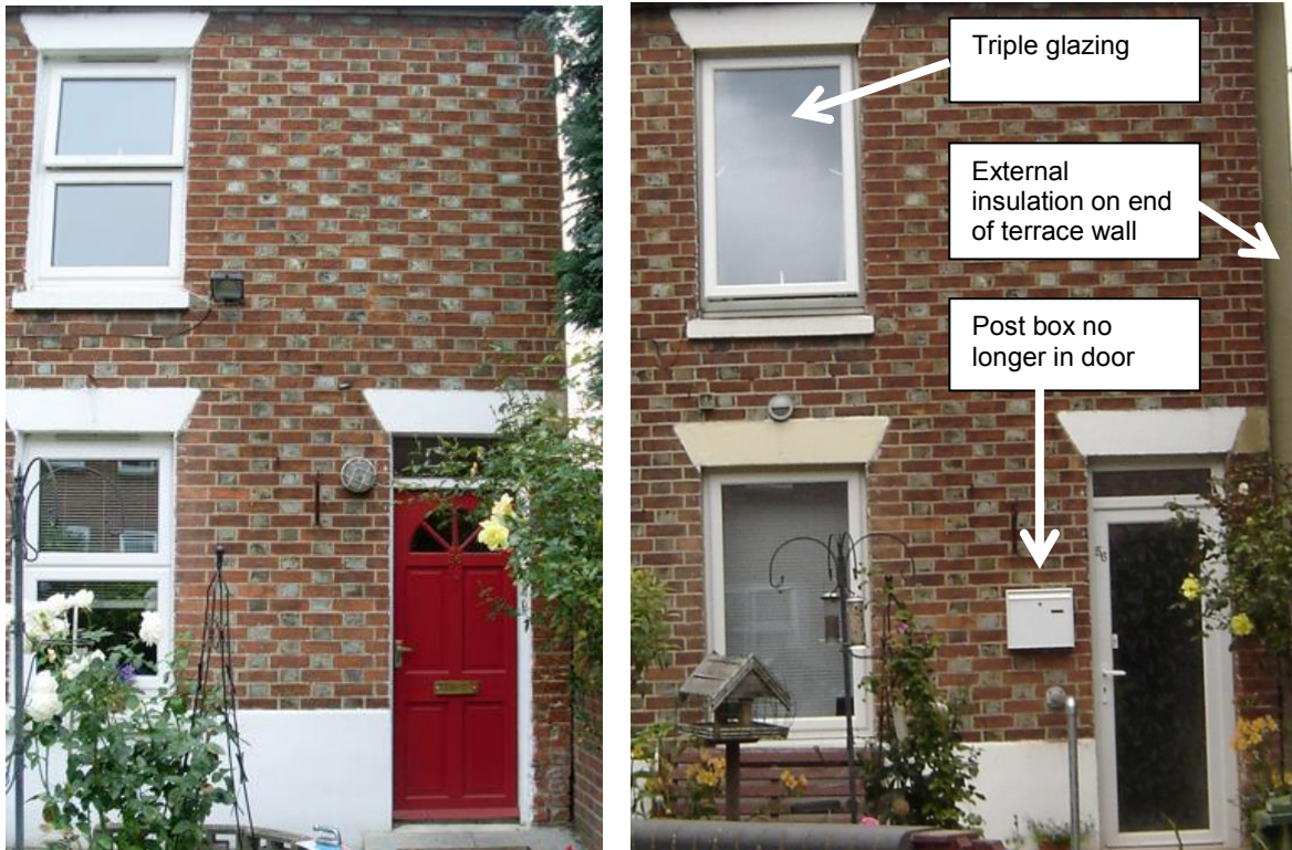
Figure 5 Front façade of Victorian house before (left) and after retrofit (right)
