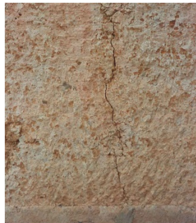
Figure 8. A vertical crack running across the full height of a wall of a rammed earth house in Mostefa Ben Brahim. Note the crack passing through the filled holes of the shuttering crosspieces.
