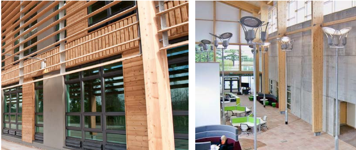
Figure 3 Exterior detail (left), three story atrium/exhibition hall (right)
