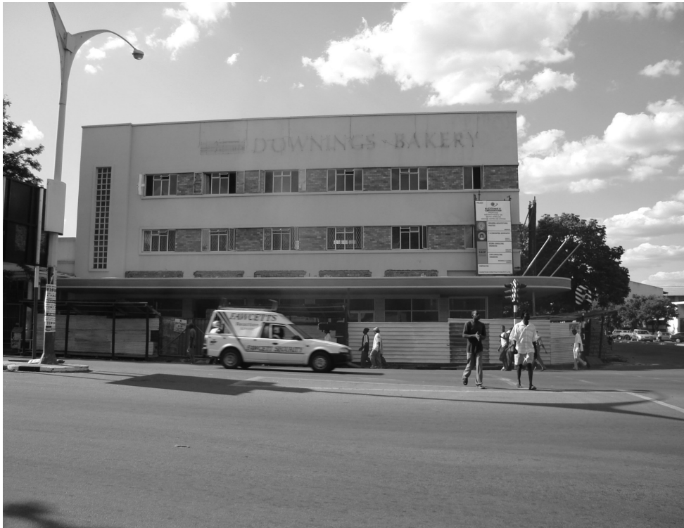
Figure 4.3 Repair and alterations April 2006; formerly Downings Bakery building to be Bulawayo HQ for the mobile phone company ECONET Pvt (Ltd). Corner of Robert Mugabe and Leopold Takawira Avenue (facing north east). Photograph courtesy of B Mbiba.
