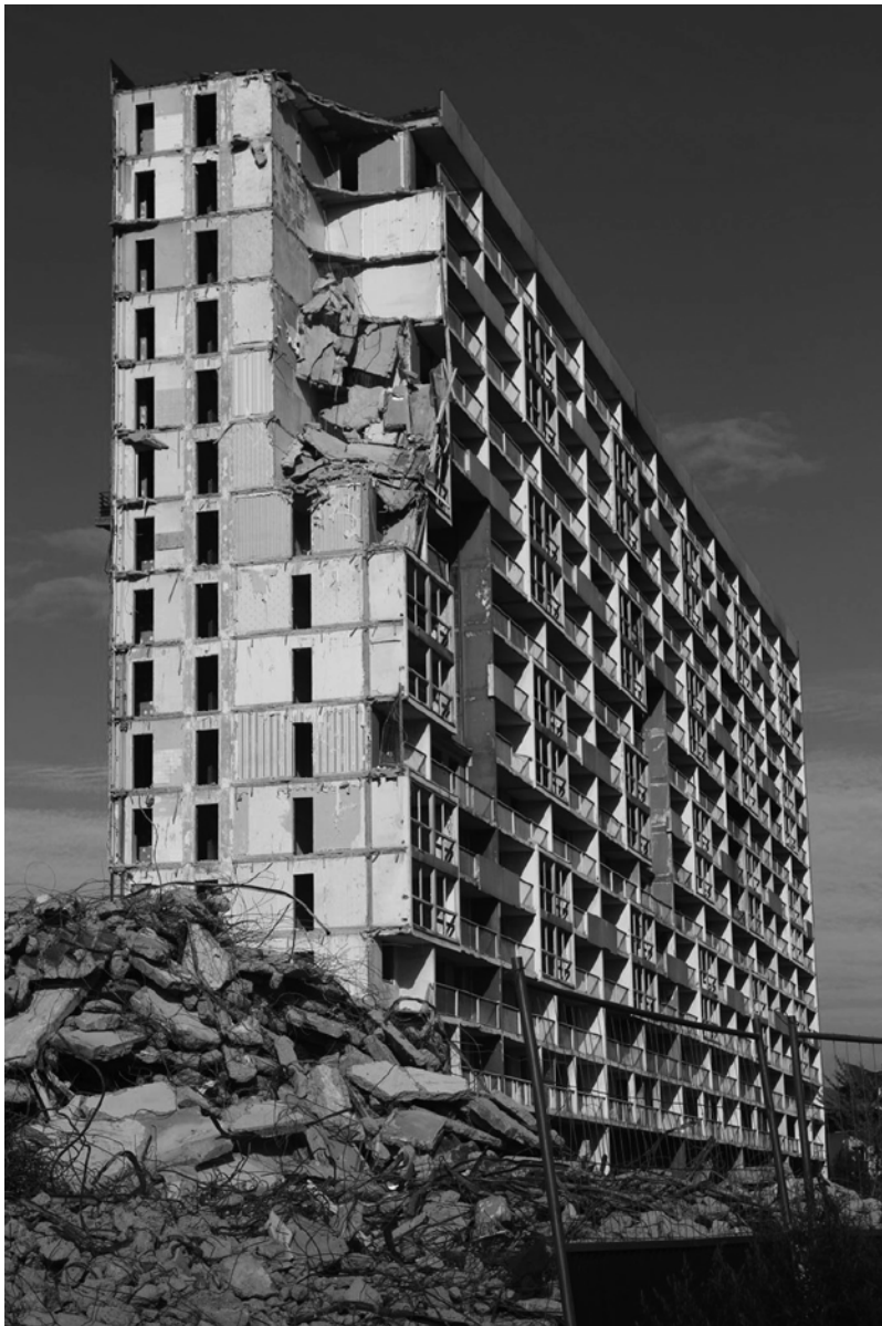
Figure 21.2 Demolition of the Balzac Tower, France Source: Diego BIS. 2011. Creative Commons 2.0.
