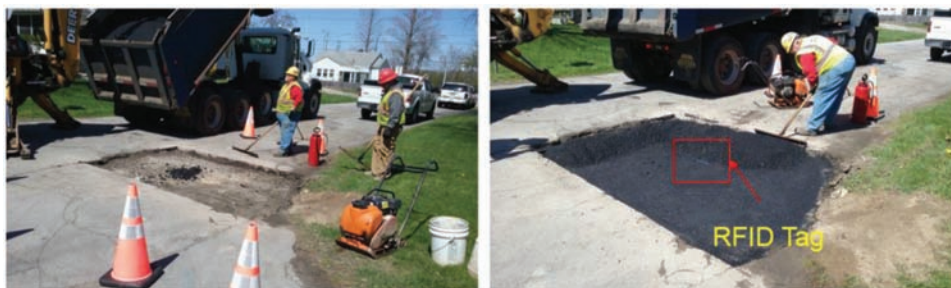
Figure 5.9 RFID tag being installed in a utility cut patch.
