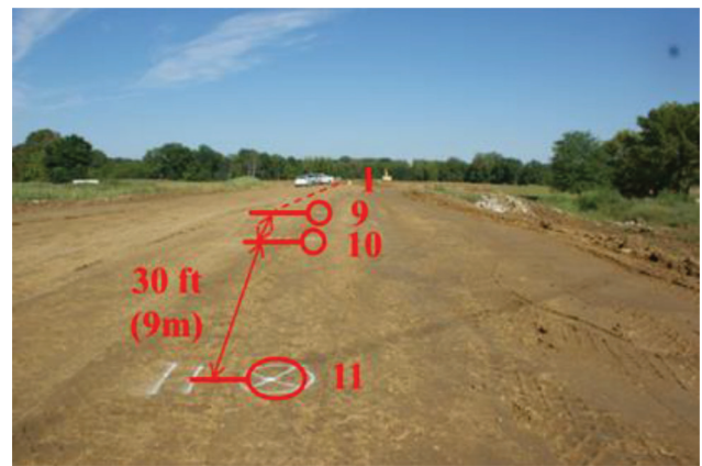
Figure A.3.9 View of the SR 641 site.
