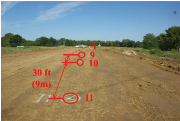
Figure 2.9 View of the SR 641 site.
