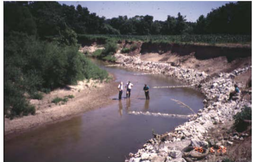
(b) Bendway Weirs in Combination with Longitudinal Peaked Stone Toe Protection
