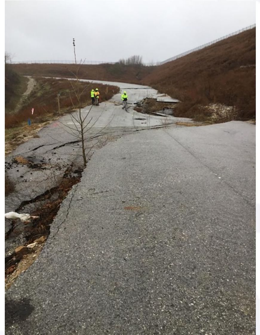
Airport Road(2018). Orange County, Indiana
