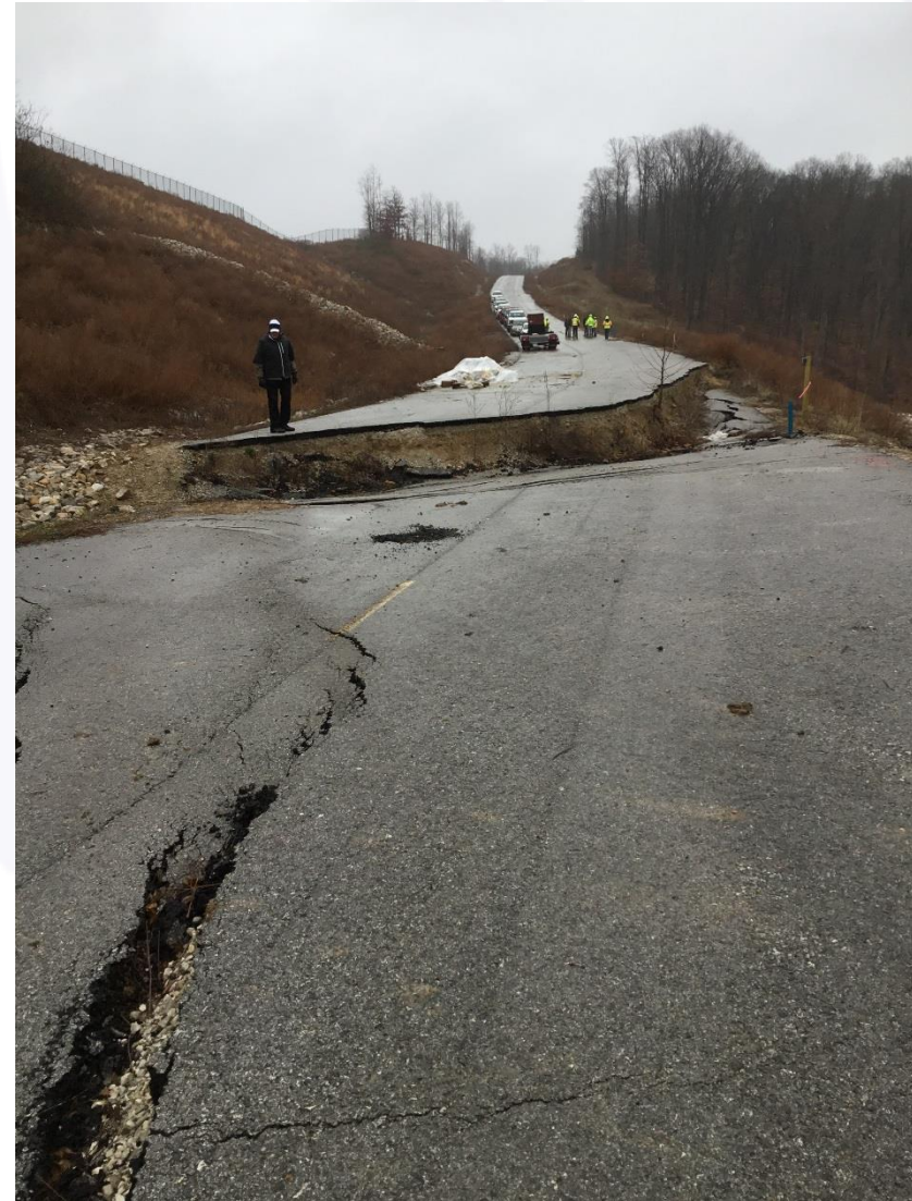
Airport Road(2018). Orange County, Indiana
