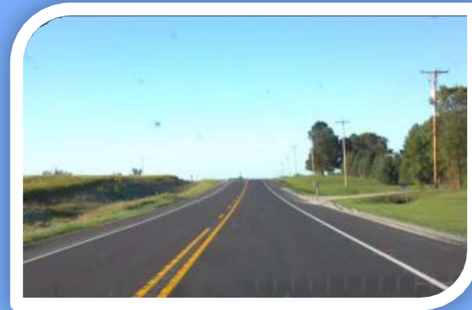
Photo Source: FHWA
