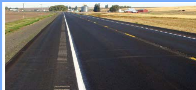
Shoulder rumble strips and center line rumble stripes are installed on this roadway.
