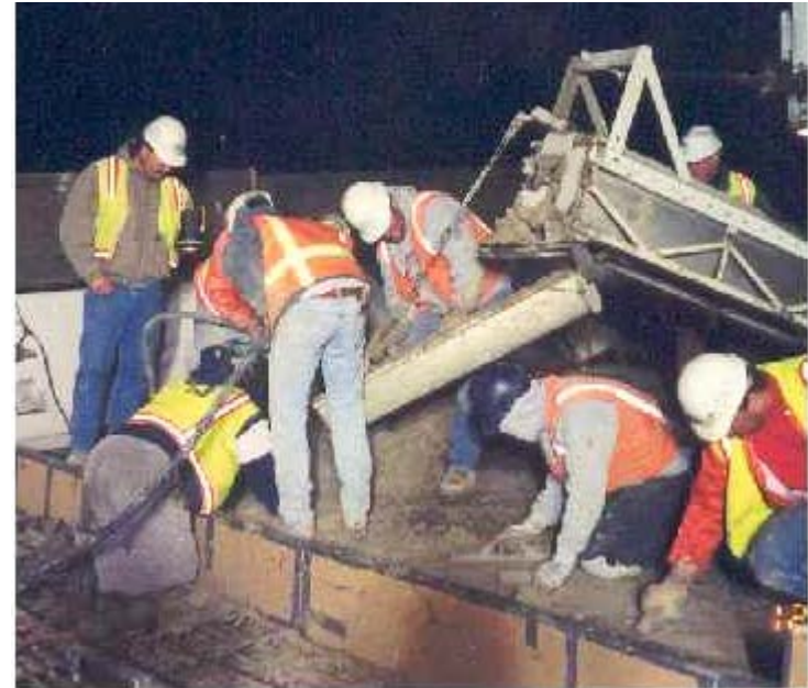
Concrete Placement Using a Mobile Mixer
