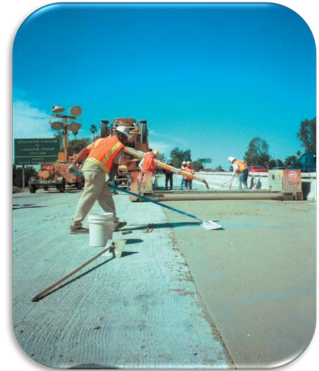
Crews Placing a Two-Mile Section of the 210 Freeway, 1999
