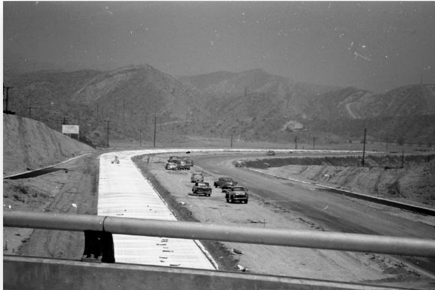
Palmdale, CA – Still in Service
