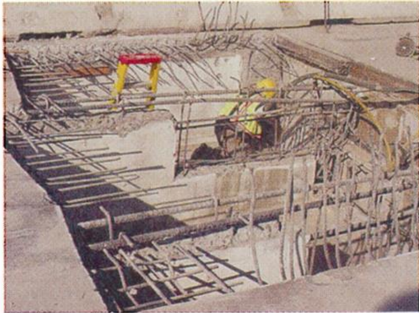
Rapid Set® Saved 7 Days of Repair Work Required Low Shrinkage
