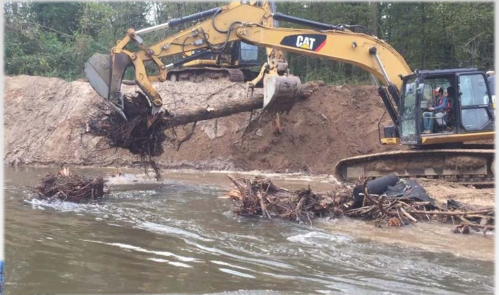
Toe wood installation along Yellow River near Knox, IN
