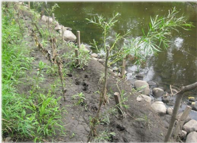
Photo courtesy of City of Golden Valley, 2018
