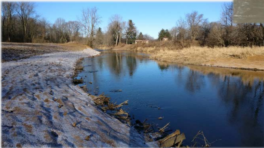
Poor initial establishment of vegetation due to timing along Yellow River near Knox, IN
