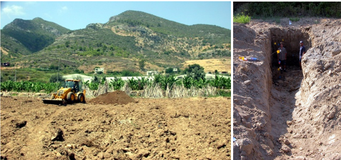
Figures 21-22: View of location of Trench H in the Kaledran river basin (left); View of excavated Trench F (right)
