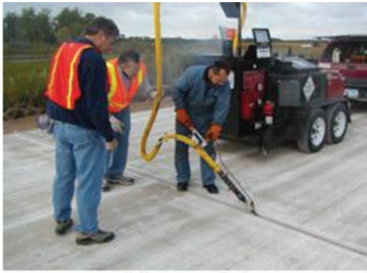
Joint Resealing a
