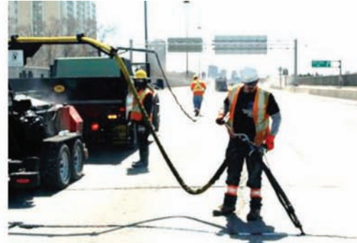
Concrete Deck Crack Sealing b
