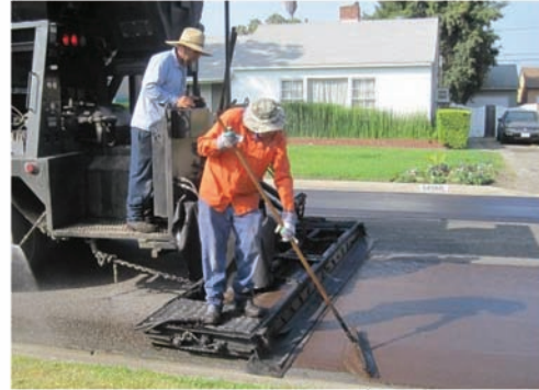
Slurry Sealing d
