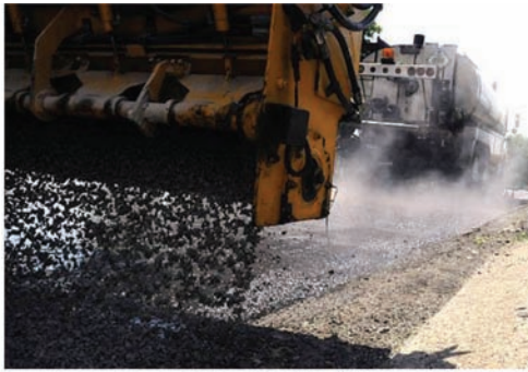
Chip Sealing a
