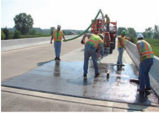
Concrete Deck Sealing a
