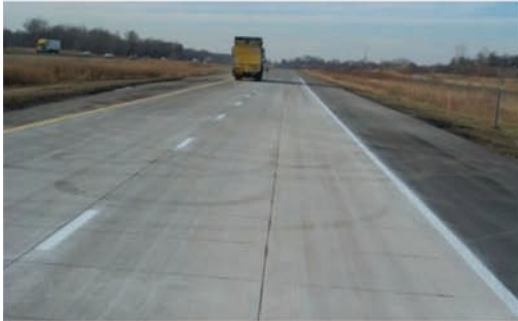
Bonded Thin-Concrete Overlays e
