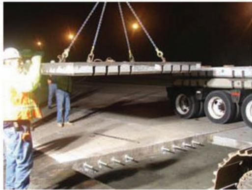
PCCP Patching c
