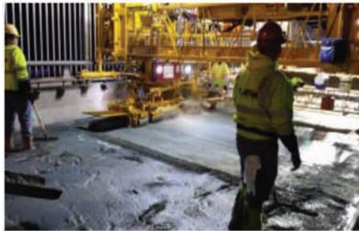
Latex-Modified Concrete (LMC) Overlay c
