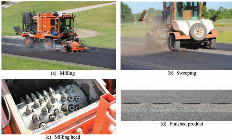
Figure 4.2 Sinusoidal rumble strip construction on June 8, 2016.
