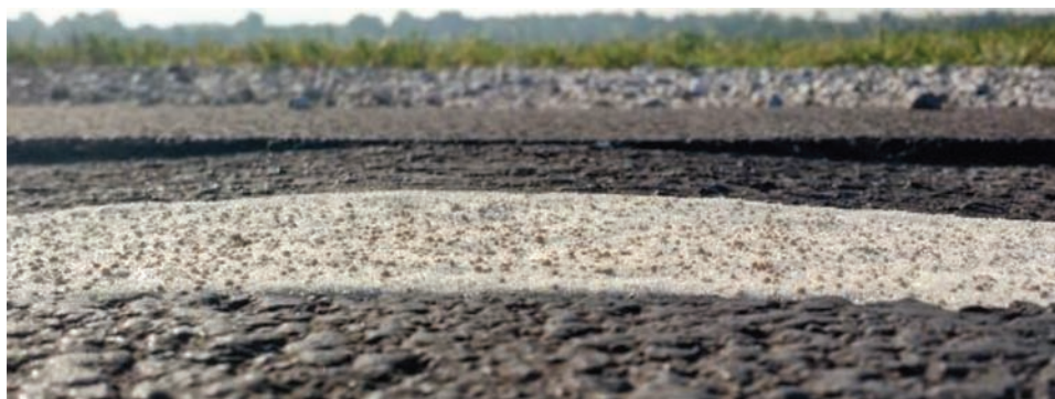
Figure 7.2 Close-up view of thermoplastic marking on sinusoidal rumble strips.
