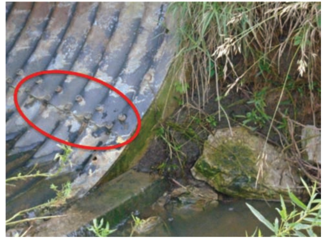
Figure 5.2 Arranged bolt pattern in longitudinal seam.
