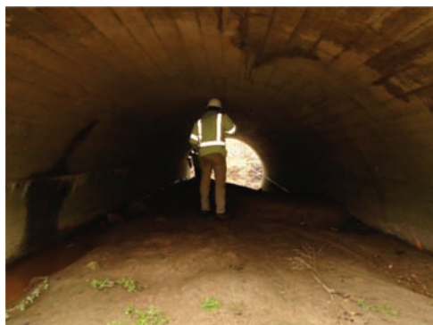
Figure 6.1 Field inspection of the northeast arch.
