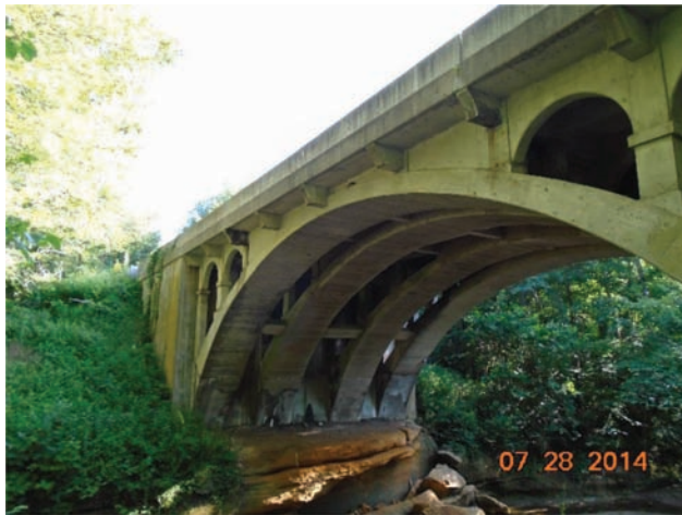
Figure 8.1 Roaring Creek Bridge.
