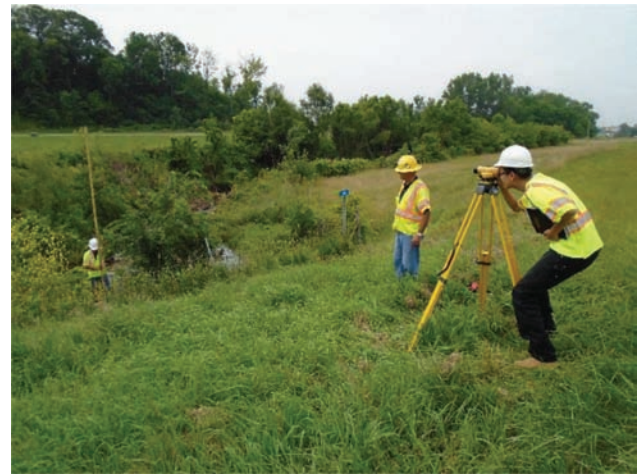
Figure 5.3 Measurement of depth of soil cover.
