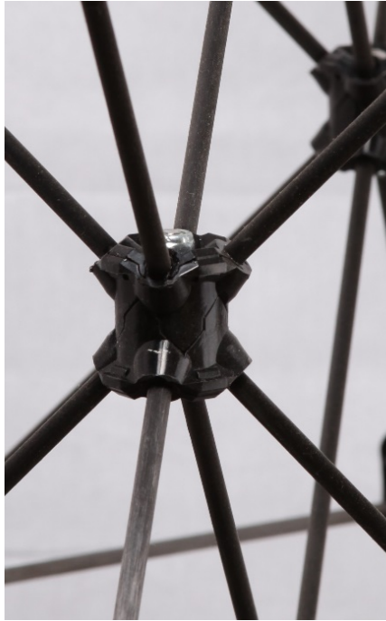
Figure 2. Detail of the node connection
