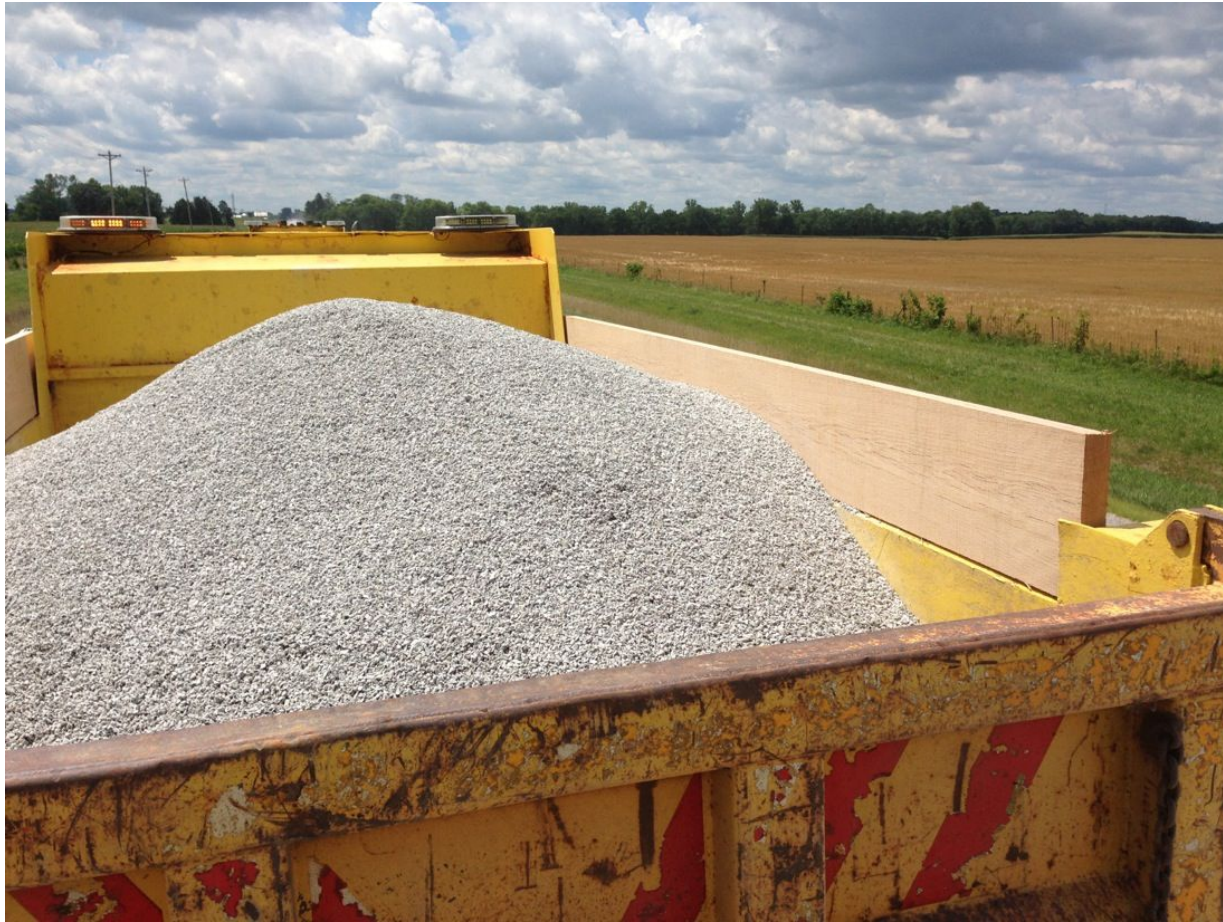
Side boards added to increase hauling capacity of trucks
