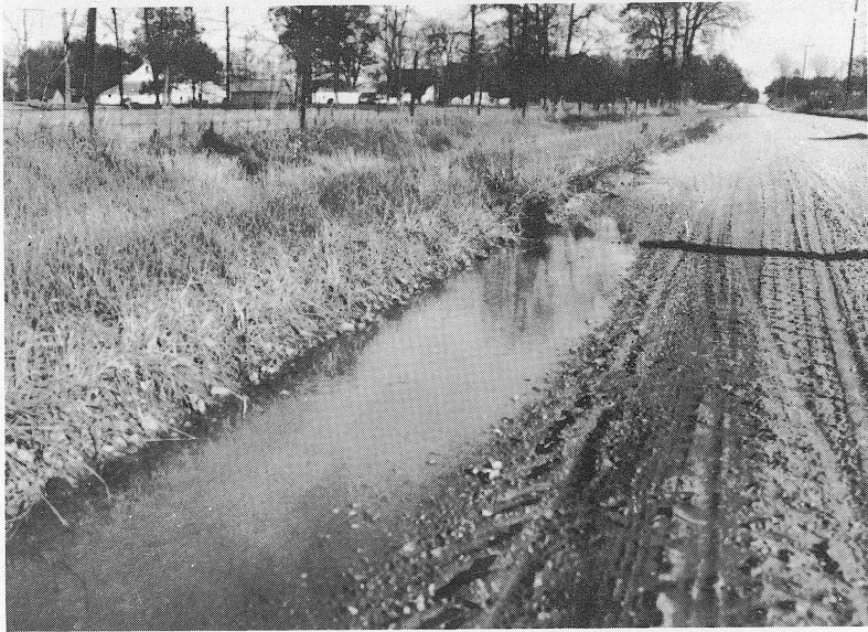
Fig. 9. This berm has no outlet. The water collected saturates and softens the roadway so that traffic creates ruts.
