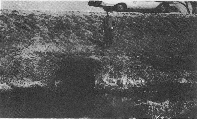
Fig. 27. The majority of county highway drainage structures are simply pipe culverts such as those shown here. (Courtesy Armco Drainage and Metal Products, Inc.)
