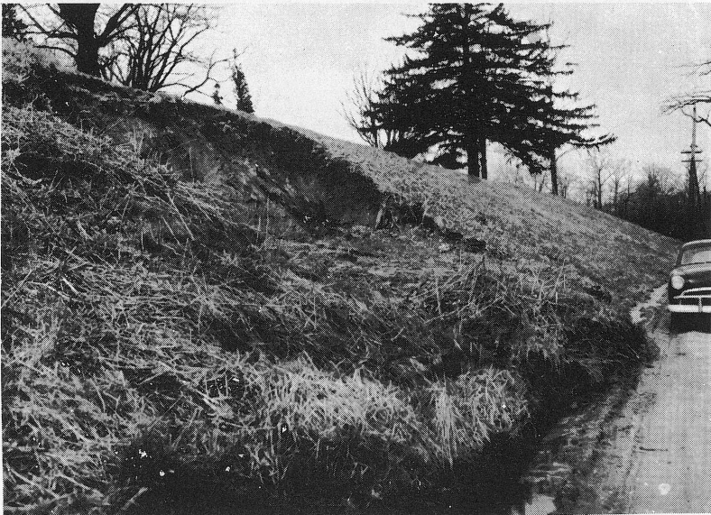
Fig. 11. No amount of grass will hold this slope which is softened by subsurface water. Subdrains must intercept the water in back of the slope to keep the soil dry.
