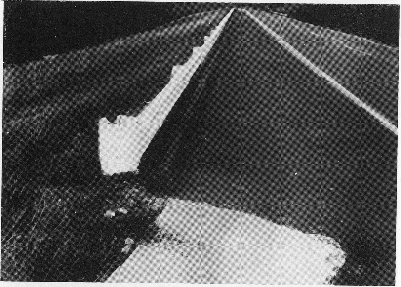
Fig. 10. This curb contains water from the long grade, so it will not destroy the side slope. Outlets both at the end of the curb and midway up the hill carry water safely to the foot of the slope.
