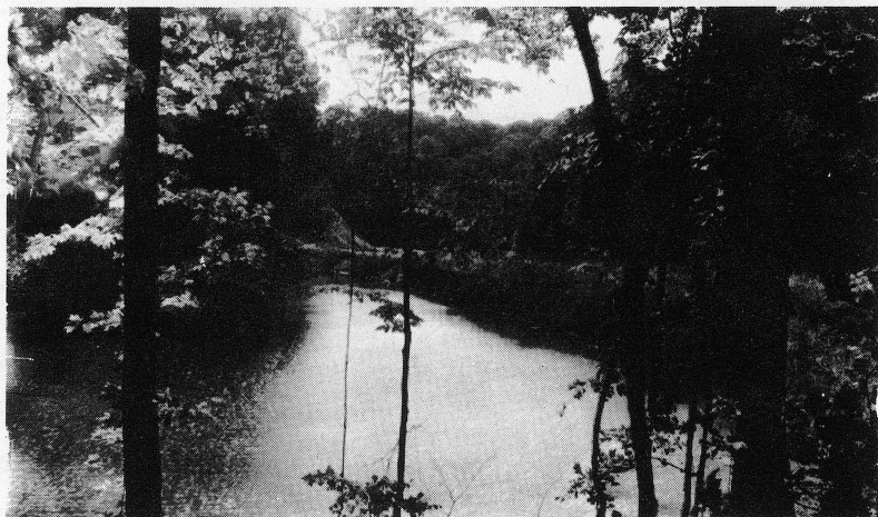
Fig. 44. This pond is created by using the highway embankment as a dam. Note the culvert outlet safely below road level at the far side of the pond.
