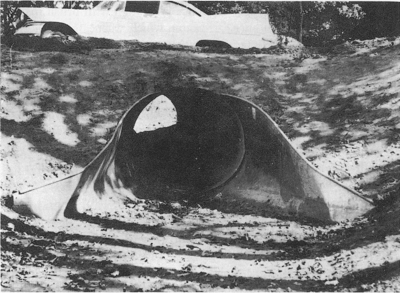
Fig. 36. A typical standard flared end section will improve entrance conditions and protect streambed and embankment from erosion. (Courtesy Armco Drainage and Metal Products, Inc.)
