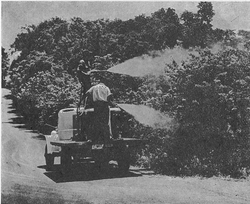
Fig. 8. Tall dense foilage, as shown here, may require several hundred gallons of herbicide mixture for both sides of a mile of road.
