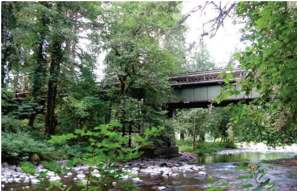
Figure 2-1 North Fork Mollala River Bridge, Oregon (OBEC, 2012)
