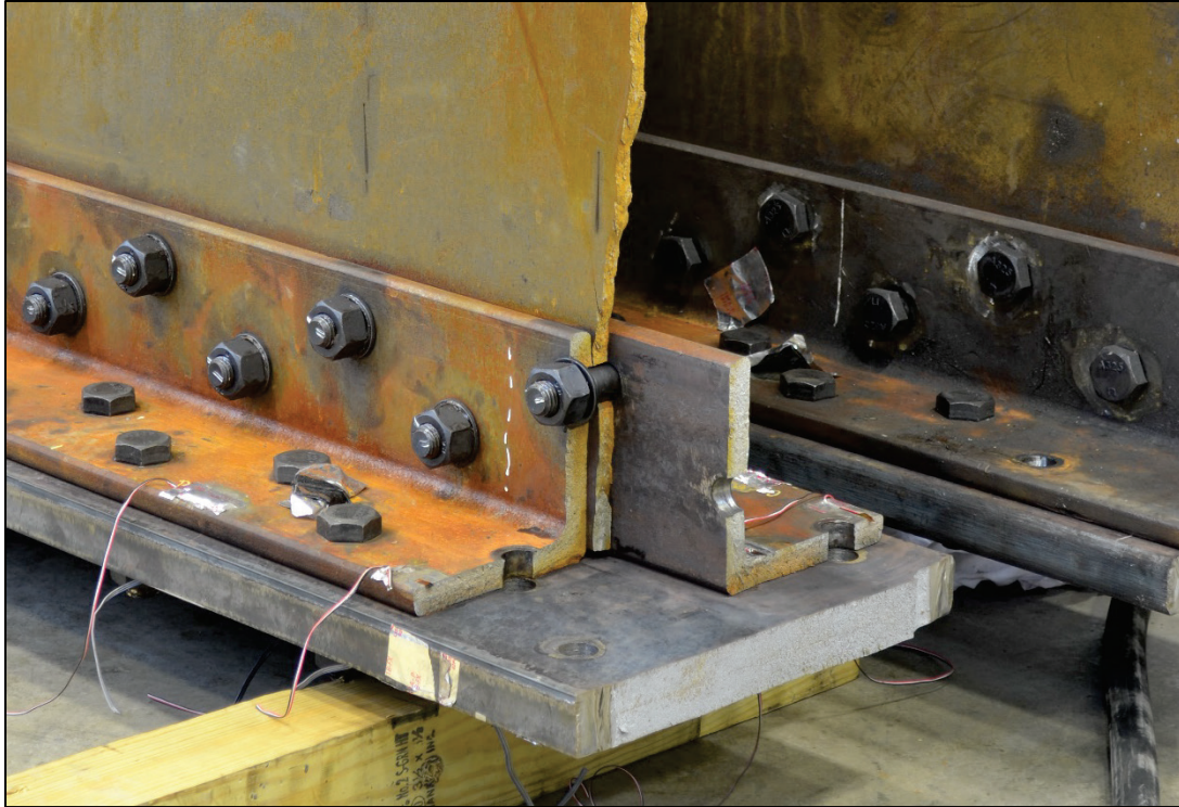
Figure 3-72 Specimen 36-5 south fracture surfaces
