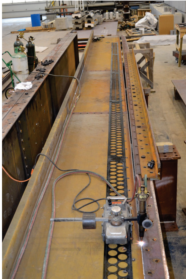
Figure 3-66 Specimen 30-1 web plate fabrication
