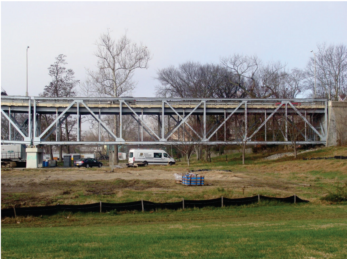
Figure 2-8 Approach span of Milton Madison Bridge, Indiana
