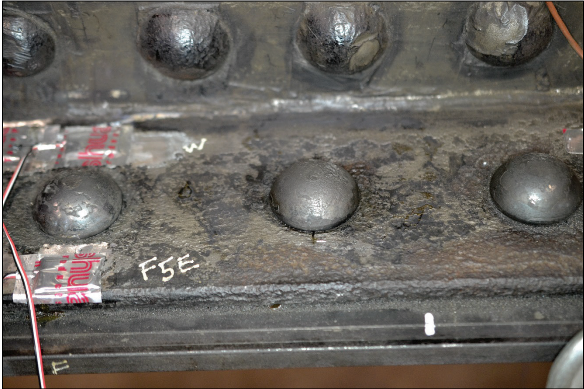
Figure 3-37 Crack growth from Specimen 23-3 hole notch
