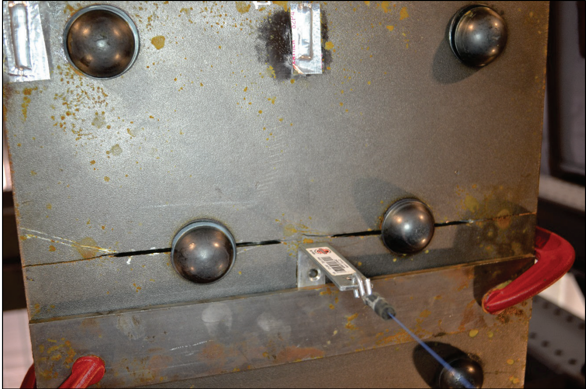
Figure 3-45 Specimen 46-3 fractured cover plate (from below)
