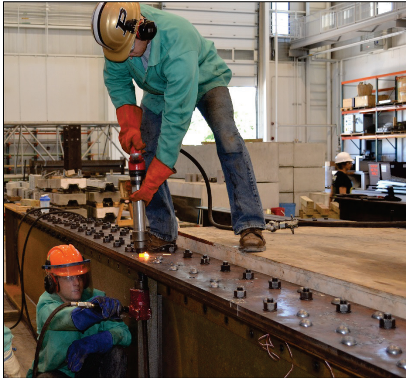
Figure 3-59 Specimen 36-3 fabrication: riveting cover plates
