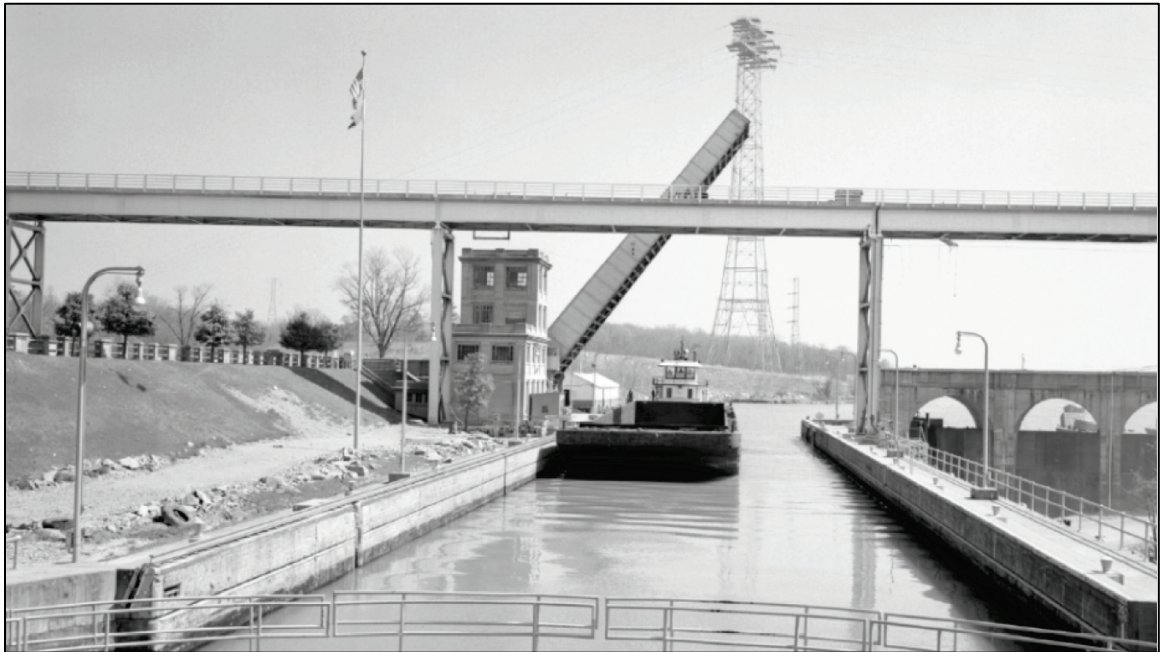
Figure 3-14 Wilson Dam Bascule Bridge in raised position in the background, 1958 (Williamson, 2012)
