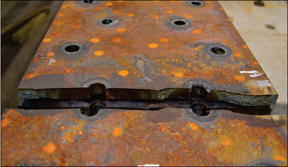
Figure 3-50 Specimen 36-1 fractured bottom flange components (bottom view)
