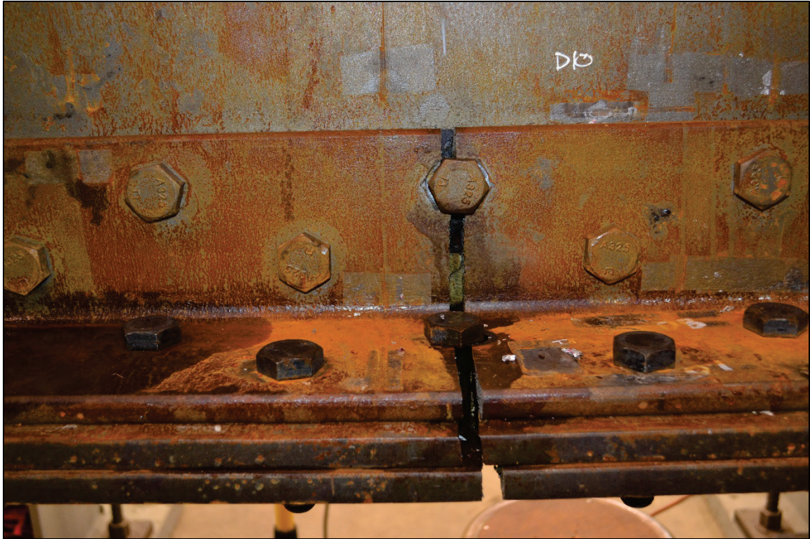
Figure 3-49 Specimen 36-1 fractured bottom flange components (east side)
