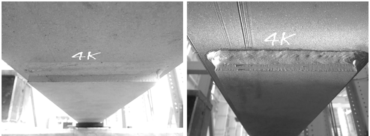
Figure 3.10a, Figure 3.10b: Cover Plate Fillet Weld Toe Before and After UIT
