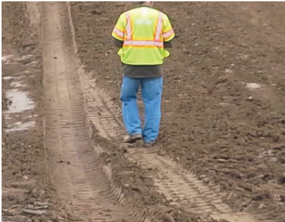
Figure C.4 Four-inch rutting @ approximately 509+00.
