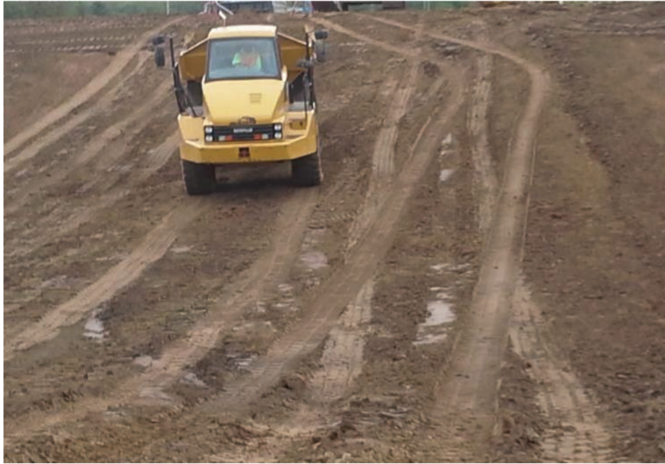
Figure C.3 No rutting at starting station.
