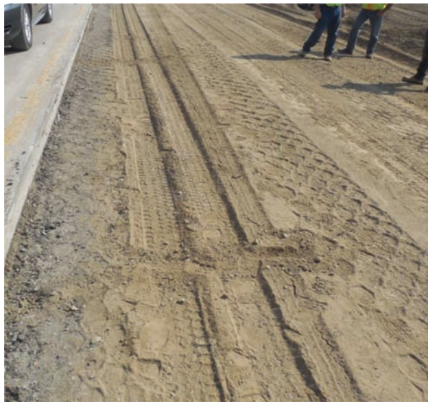
Figure C.11 Beginning of proof roll with no rutting.
