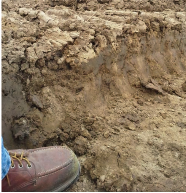
Figure C.5 Eight-inch rutting @ approximately 508+50.
