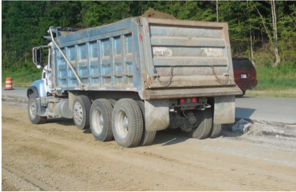
Figure C.11 Beginning of proof roll with no rutting.
