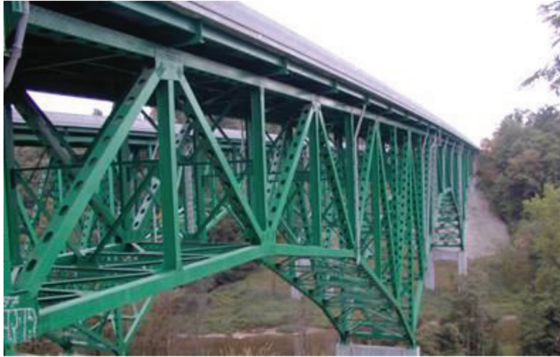
Figure 1.1 Truss diagonal showing typical hand hole details.
