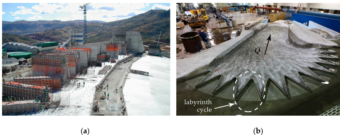
Figure 1. Examples of arced labyrinth weirs: (a) Maguga Spillway in Swaziland during construction, and (b) the physical model of Isabella Spillway to be built in California, United States of America (USA). Photos courtesy of D. van Wyk (a) and B. Tullis (b).
