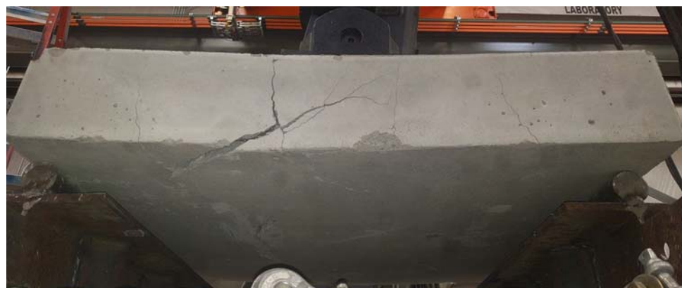
Figure 5-7 Cracks 1/2 inch (approximately 25,000 cycles)
