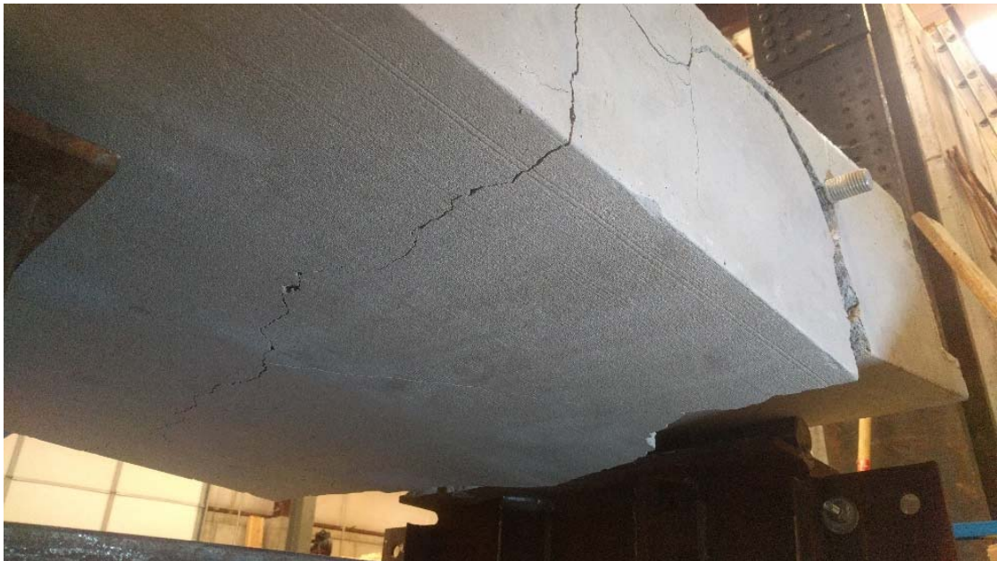
Figure 5-26 Pad after failure
