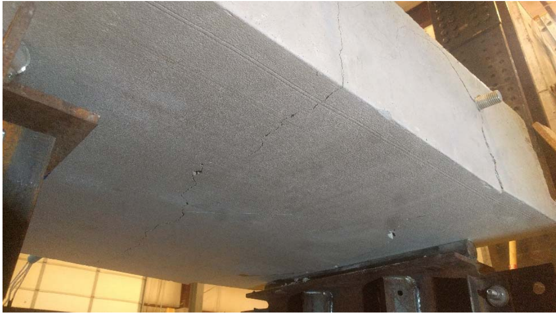
Figure 5-25 Crack 1/2 inch wide
