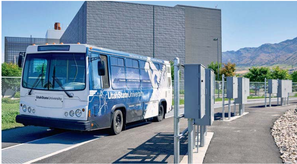
Figure 3-2 EVR Test track and Power Panels
