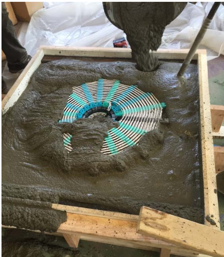
Figure 3-13 Pouring first inductor pad
