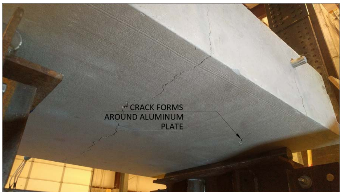
Figure 5-24 Crack 1/4 inch wide
