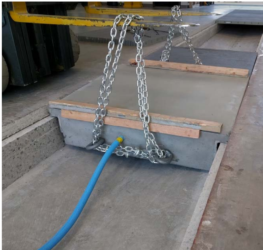
Figure 3-14 Installation of the first concrete embedded IPT coil
