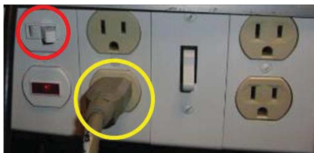
FIG. C.5. ESD power supply switch (outlined in red). This switch controls the bank of plugs to the right of it. In this image the current position is “on,” turned to the right and the CPS power supply cord is outlined in yellow. The red light (under the switch) indicates that the power supply is on and the user should take caution.
