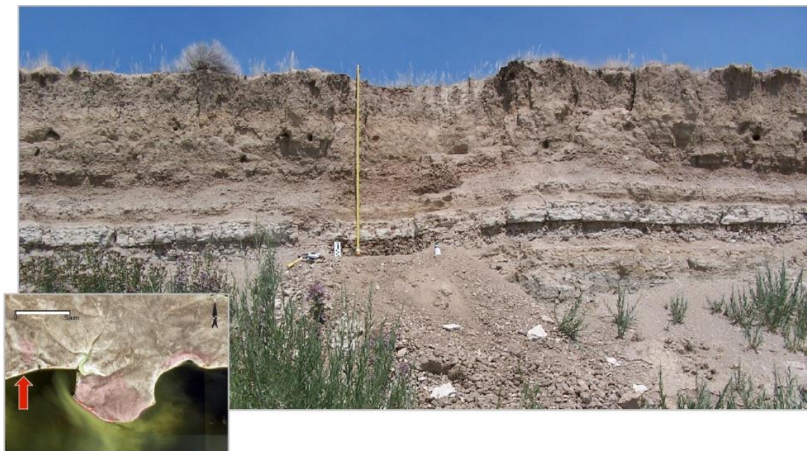
Figure 15. Overview of Profile 9, view north.
