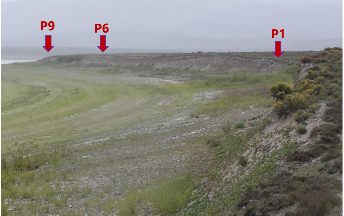
Figure 14. Overview of west end with profile locations marked. View northwest.
