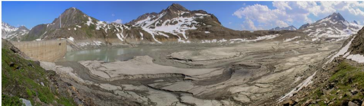
Figure 1: Aggradation pattern in Gries reservoir, Switzerland, with lowered reservoir level during construction works at the dam (on the left) on 2 July 2015 (Photo: D. Ehrbar)
