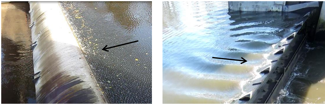
Figure 3: Left: standing waves in the headwater of a lifting gate with underflow. The waves are caused by the vibration of the spring-supported seal system. The vibration frequency is between 15 and 20 Hz. Right: standing waves in the headwater of a 42 m wide vibrating lifting gate during underflow. The bending amplitude at the midpoint of the gate is 1.6 cm and the frequency is 1.5 Hz. In Both pictures the flow direction is marked with an arrow.
