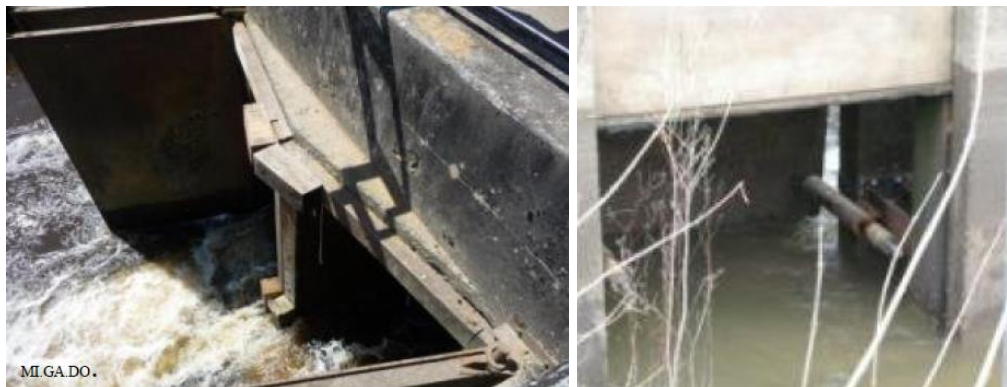
Figure 1. block on a side-hinged gate (left) and stiffener on a Top-hinged gate (right) (Lauronce et al. 2015)
