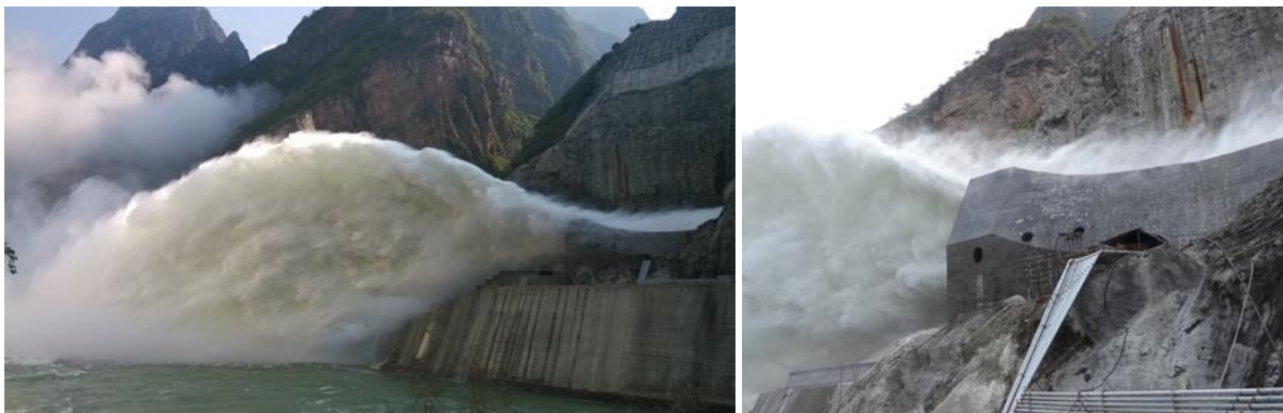
Figure 1. Ski-jump flow of leak-floor flip bucket in Jinping hydropower station.
