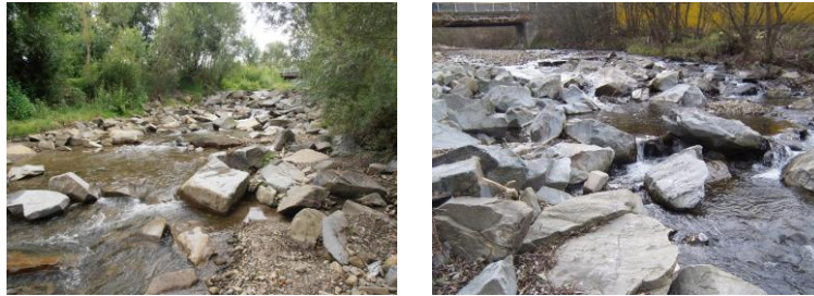
Figure 1. Boulder block ramp on Poniczanka stream: upstream view and a focus view of a ramp
