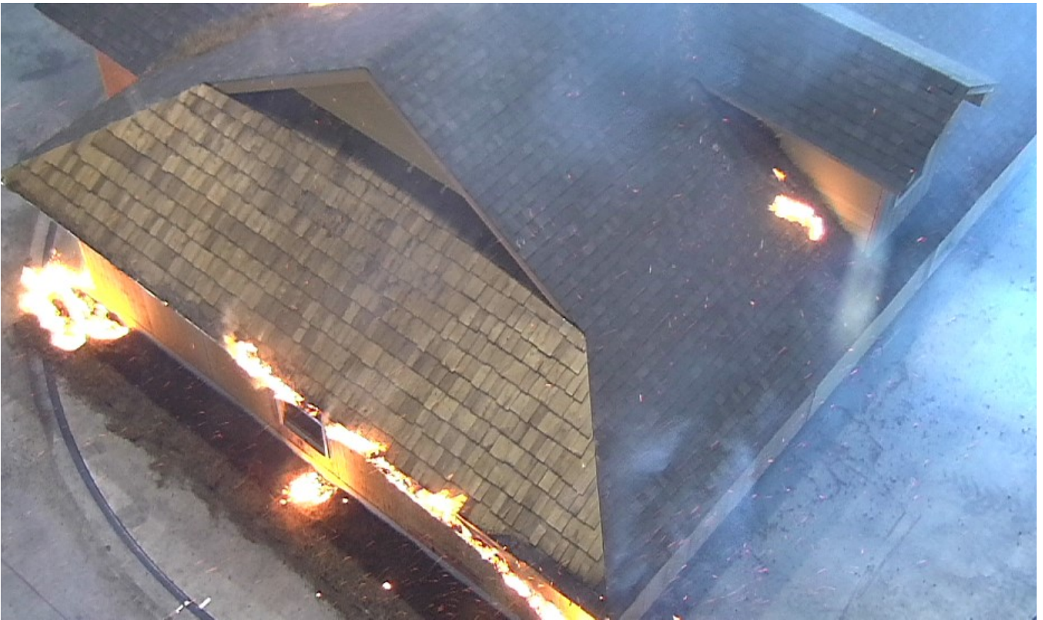
Figure 4. Burning pine needles in the rain gutters and burning pine needle debris on the roof against the dormer (on the right). This dormer is representative of vulnerability to embers that occurs on a “complex” roof, particularly at roof-to-siding intersections. Photo: Jack Cohen, USDA Forest Service and IBHS.
