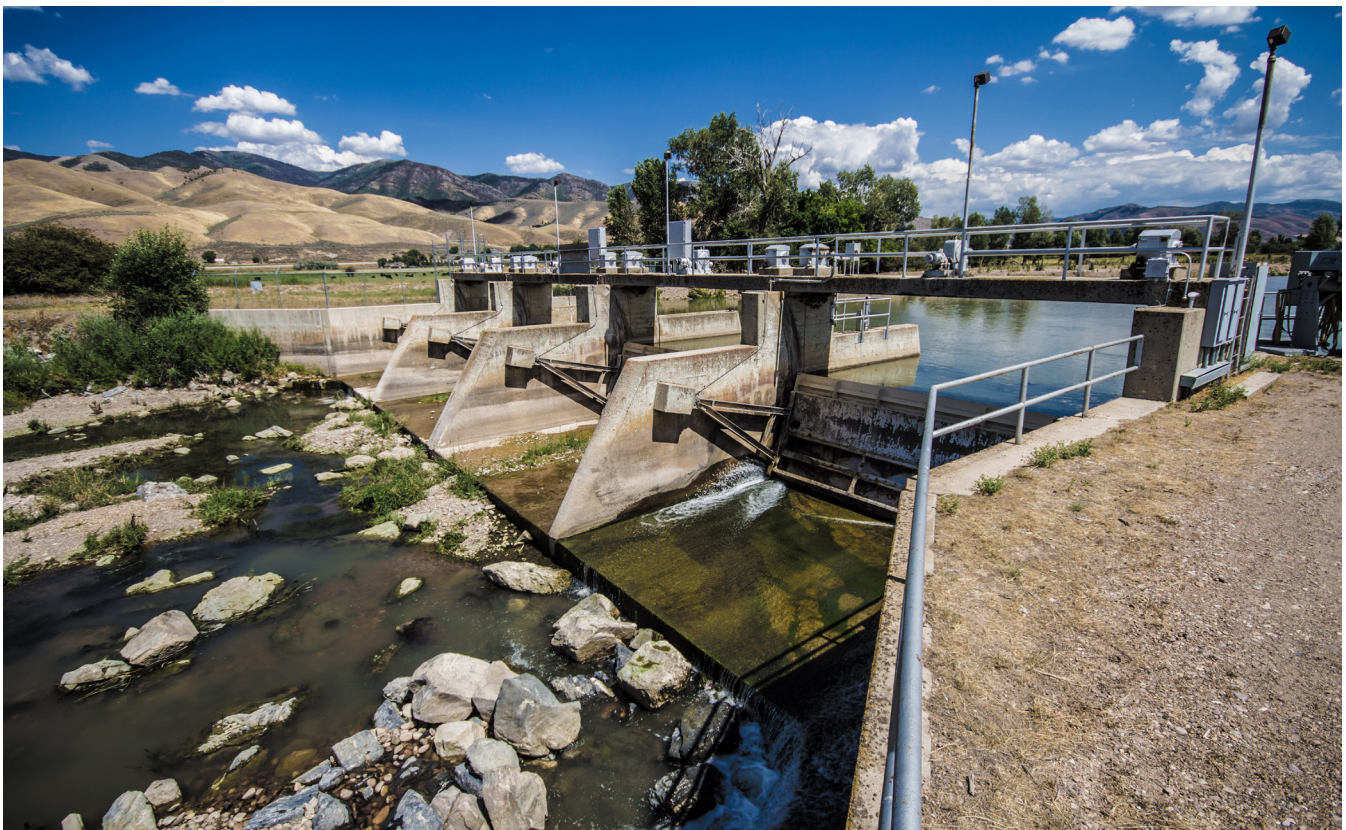
Fig 2.2: Dewatering downstream of the Stoddard Diversion.
