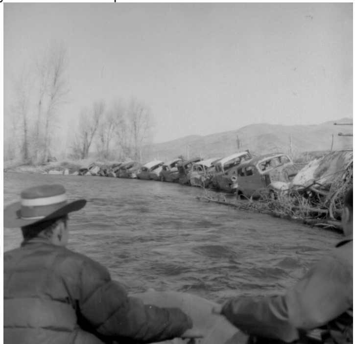
Fig 1.9: Historic photo of car bodies installed along the banks of the Weber River.
