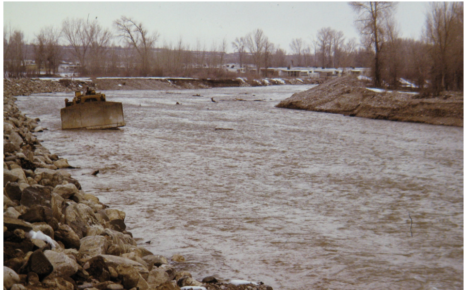
Fig 4.4: Historic Channelization of the Weber River.
