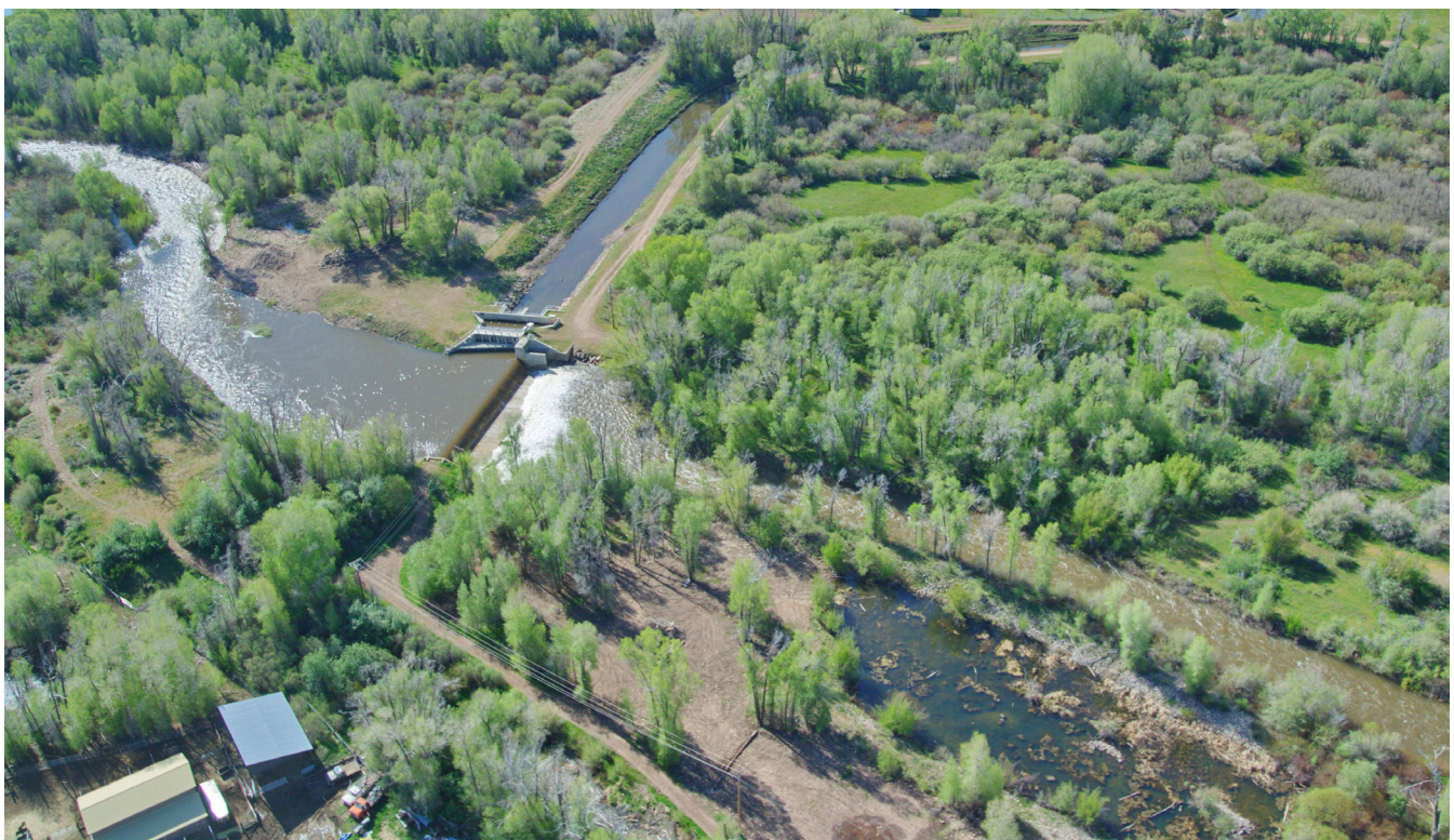
Fig 3.8: Image of the Weber-Provo diversion structure in Kamas.
