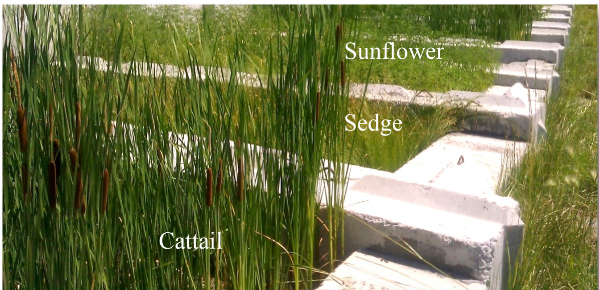
Figure 2. Vegetated treatment bays at the Green Meadows Field Stormwater Management Demonstration Site, Logan Utah.
