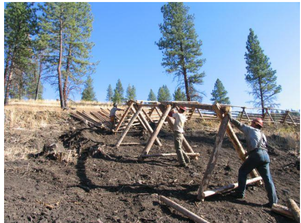
Photo 4. Buck and pole fence construction at Dovenberg demo site.
