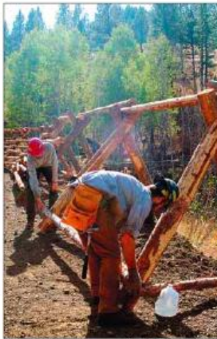
Grayback workers Don Gabbard (left) and Mat Elliott position a pole in a fence that is being built to protect a fire-damaged aspen grove.
