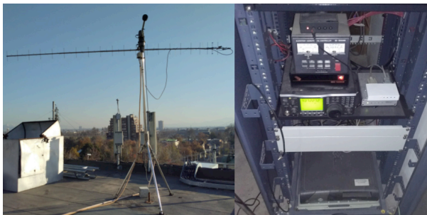
Figure 5: Ground station equipment.
