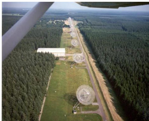
Figure 3: The Westerbork Synthesis Radio Telescope (WSRT) consisting of 14 dish-shaped antennas.
