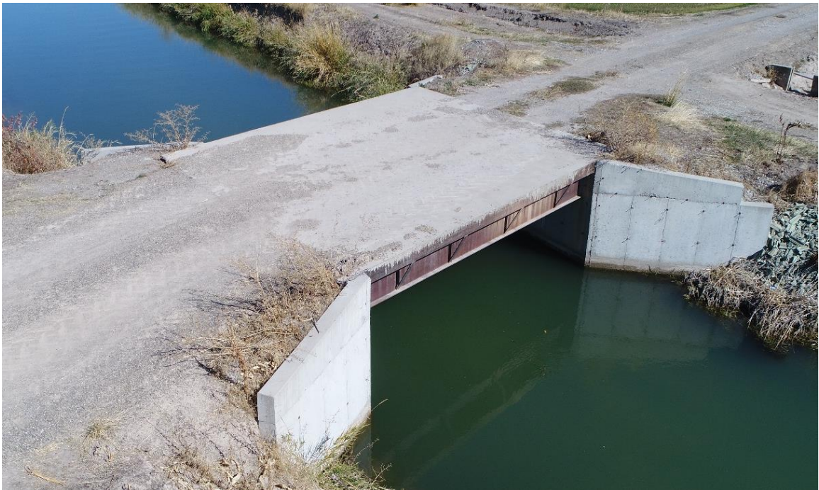
Figure 67. Photograph of the Elwood Bridge.
