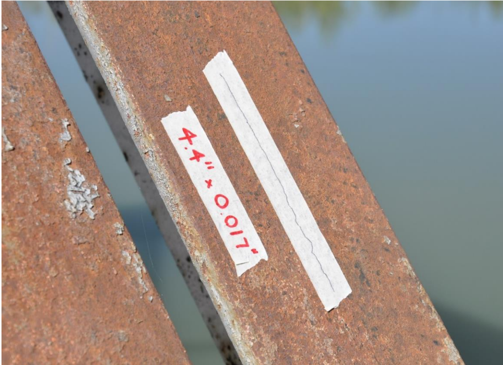
Figure 64. Artificial “crack” at the Trenton Bridge.
