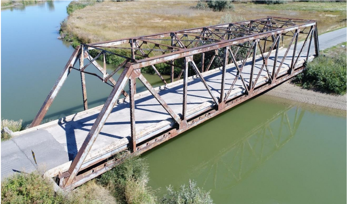
Figure 66. Photograph of the Trenton Bridge.
