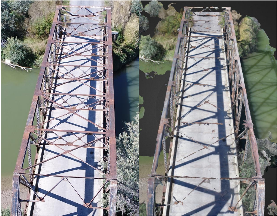
Figure 72. Comparison of Trenton Bridge trusses to DroneDeploy model trusses.
