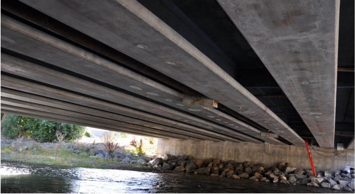
Figure 15. Underside of the Nibley Bridge.
