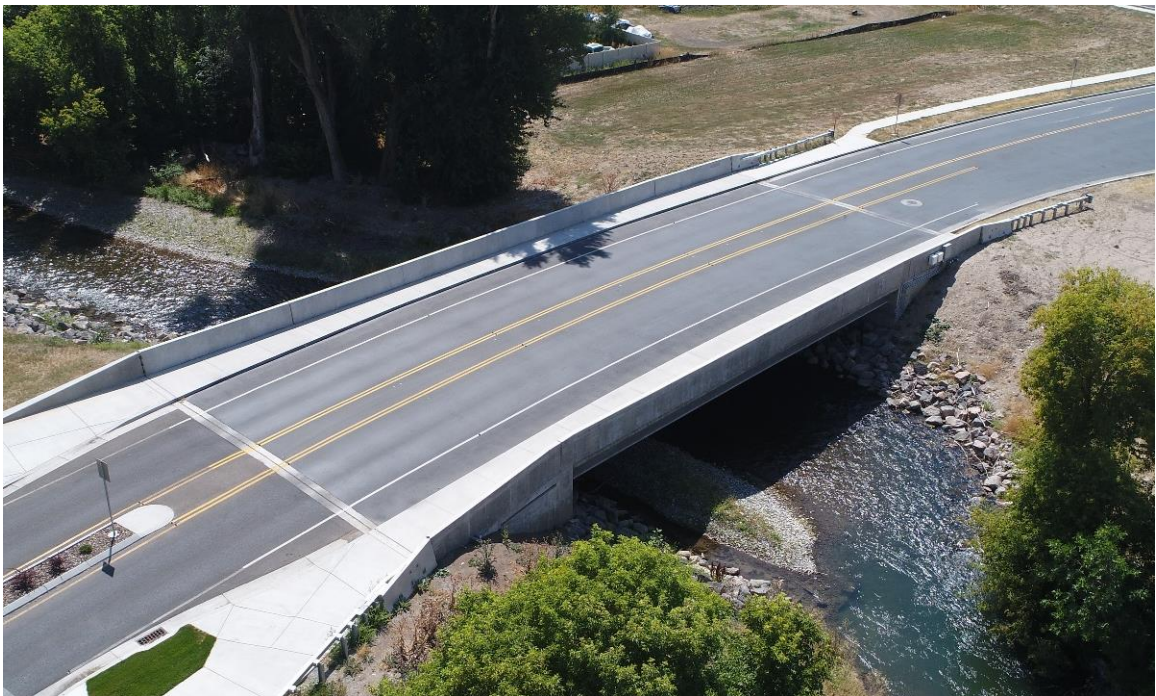
Figure 65. Photograph of the Nibley Bridge.
