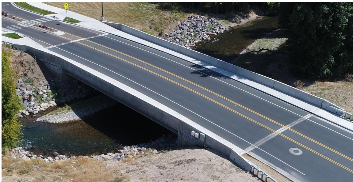
Figure 11. Photograph of the Nibley Bridge.
