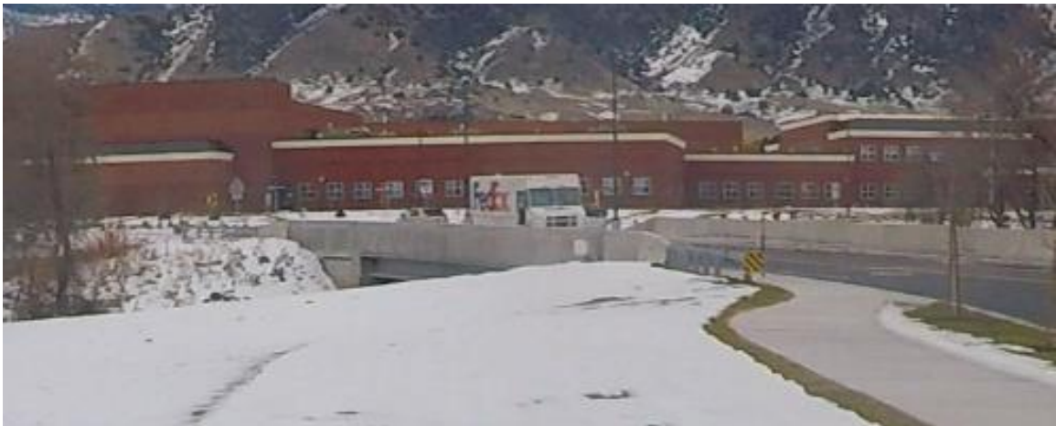
Figure 26. Still from recorded video showing a vehicle crossing the Nibley Bridge.
