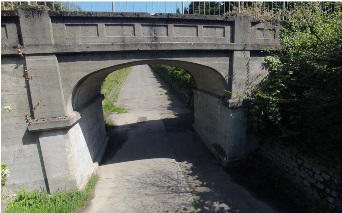
Figure 9. Photograph of Pedestrian Bridge (Lattanzi and Miller 2015).
