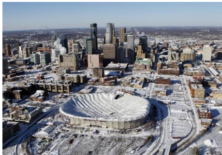
Figure 1: Minneapolis Metrodome, December 2010[8].
